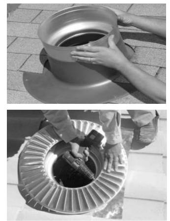
**STEP 3:** Carefully mount the top cover over the shroud and secure it with (4)  $\# 8 \times .500$ " self-tapping stainless steel screws (supplied). Use the supplied roof caulk to seal any loose shingles as well as the areas where the slits were cut, and around the top and shingles over the flashing.
