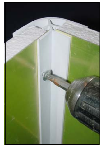
FIGURE 8: INSTALLING CORNER CONNECTORS
