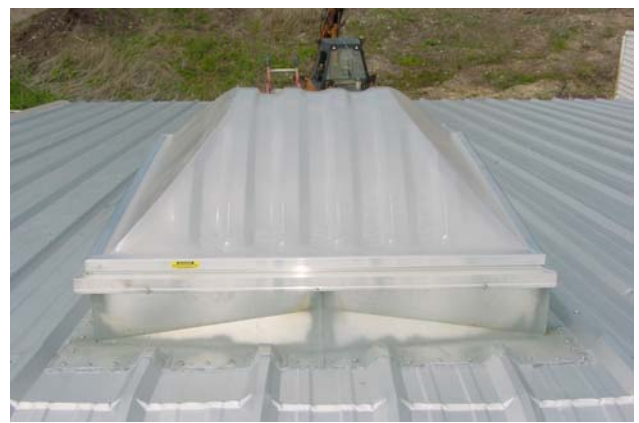
Factory built metal roof curb, secured in place, with built-in diverter or cricket on the peak side of roof
