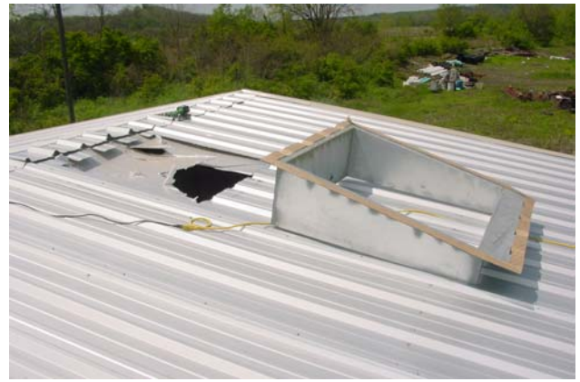
Factory built metal roof curb (pictured upside down with gasket installed) ready to be installed on metal roof
