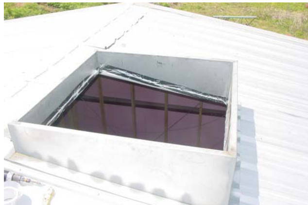
Factory built metal roof curb in place, ready for fasteners
