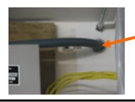
Left: Close up of Parans Optical Cable bundle entering the building through 1.5" conduit
