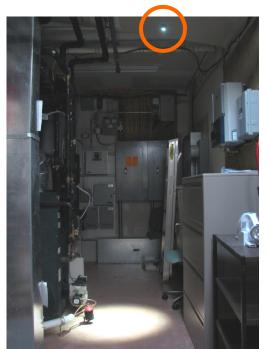
Left: In the mechanical room a Parans L3 Luminaire was installed. This is a small spot light type fixture. (see the orange circle around fixture which is creating the spot light on the floor) This L3 is fed by one fiber optic cable, 10 meters long.
