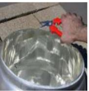
STEP 9: Remove protective film from Light Tube and install Dome Assembly (Item # 1). Secure to Flashing with No.8 x 3/8" Stainless Steel Screws (Item # 2). IMPORTANT: Do not apply ANY silicone around Dome Assembly for it can create and keep condensation inside skylight. Finish roof installation by sealing around Flashing and gluing any loose shingles with supplied Roof Caulking.
