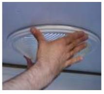
Do NOT leave the protective film exposed to the sun or it may become difficult to remove. Also avoid placing the tube on or near combustible material once the protective film is removed due to the chance of fire if exposed to sunlight.
