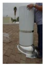
**STEP 8:** On roof, trim Light Tube (if necessary). Flush with top of Flashing using Tin Snips. Or score outside of Light Tube with a utility knife at top level of Flashing and push against it to cut.
