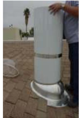
**STEP 7:** Bring Light Tube down flush to the Trim Ring. Do not go lower; it can be 1/4" higher from Trim Ring. Fasten Light Tube to Trim Ring with 3 or more No.8 x 1/2" Self-Drill Sheet Metal Screws (**Item #8**). **DO NOT OVER TIGHTEN.** Keep Light Tube as round as possible against Dust Seal.
