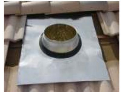
**STEP 4:** Apply Roof Caulking at any gaps created between aluminum and EPDM Rubber while contouring Aluminum Skirt to tiles. Paint to match color of roof. To complete installation, follow **STEPS 4 through 10**, same as for shingle roofs.
