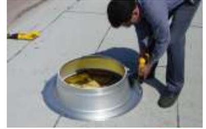
**STEP 2:** On roof, locate pre-drilled hole. Use supplied roof template to mark circumference of hole for Flashing. Cut hole (**DO NOT CUT ANY FRAME MEMBERS**). Apply two ½” thick beads of High Quality Roof Caulking (supplied) on under side of Flashing. Secure to roof using No.8 x 2” or longer Stainless Steel Screws (**Item # 5**).
