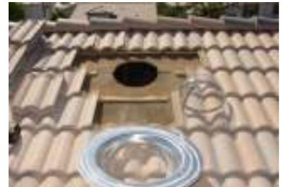
**STEP 3:** Replace tiles at lower side of Flashing. Place Aluminum Skirt with EPDM Rubber (supplied for tile roofs) over Flashing as shown. Adjust Aluminum Skirt to fit profile of tiles. Cut rest of tiles to fit around Flashing as needed and apply Roof Caulking wherever may be needed.
