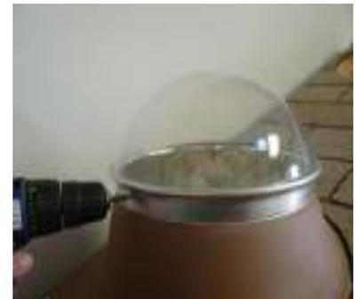
**STEP 10:** Finally, remove any protective film from inside Light Tube and install Ceiling Deco-Ring (**Item # 13**) with Light Diffuser (**Item # 12**). Install by aligning stand offs with keyholes and twist right (clock wise) until ring stops. **If Ceiling-Deco Ring ever needs to be removed for cleaning, twist left (counter clock wise), remove, clean and install back to original position.**
