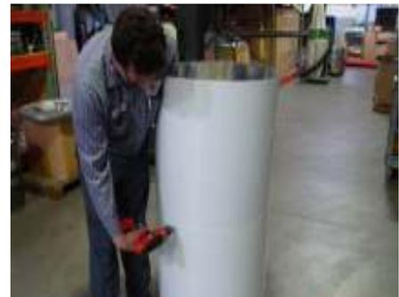
**STEP 6:** Once Light Tubes are assembled, these can be installed from roof. Crimped side should go in first for easier install. Elbows can be used for obstructed attics.
