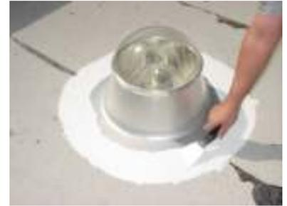
**STEP 3:** Apply a 4” wide reinforcement fabric around perimeter of Flashing and High Quality Roofing Mastic (not supplied) to double seal any potential water leakage. To complete installation, follow **STEPS 4 through 10**, same as for shingle roofs
