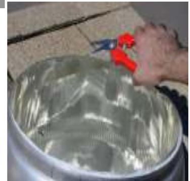
**STEP 9:** Remove protective film from Light Tube and install Dome Assembly (**Item # 1**). Secure to Flashing with No.8 x 3/8" Stainless Steel Screws (**Item # 2**). **IMPORTANT: Do not apply ANY silicone around Dome Assembly for it can create and keep condensation inside skylight.** Finish roof installation by sealing around Flashing and gluing any loose shingles with supplied Roof Caulking.
